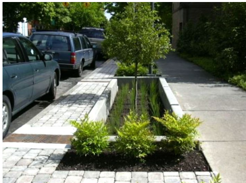
Curbside planting with bioswale
