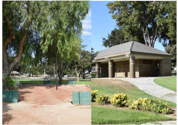
Horseshoe Pits / Restroom Building
