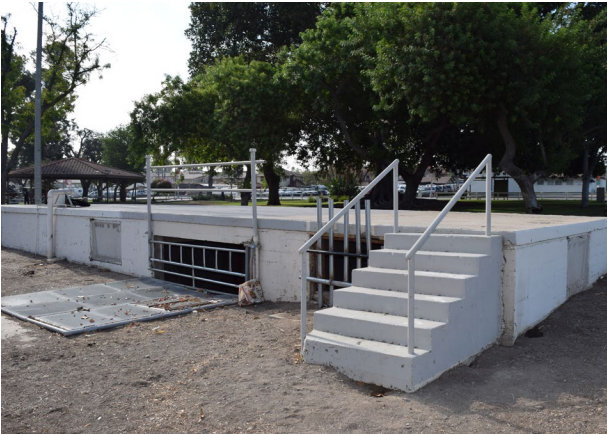
Former Pump Building
