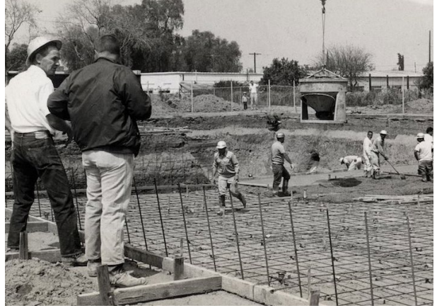
New swimming pool construction (c. 1967)
